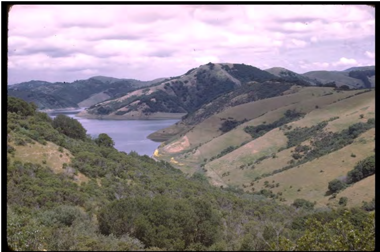
Upper San Leandro Reservoir Photo Credit: Charles Webber, California Academy of Sciences © 2002
