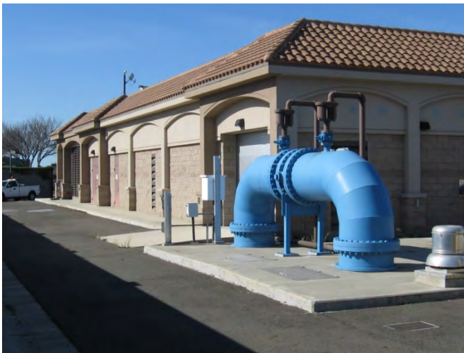
Skywest Pump Station
