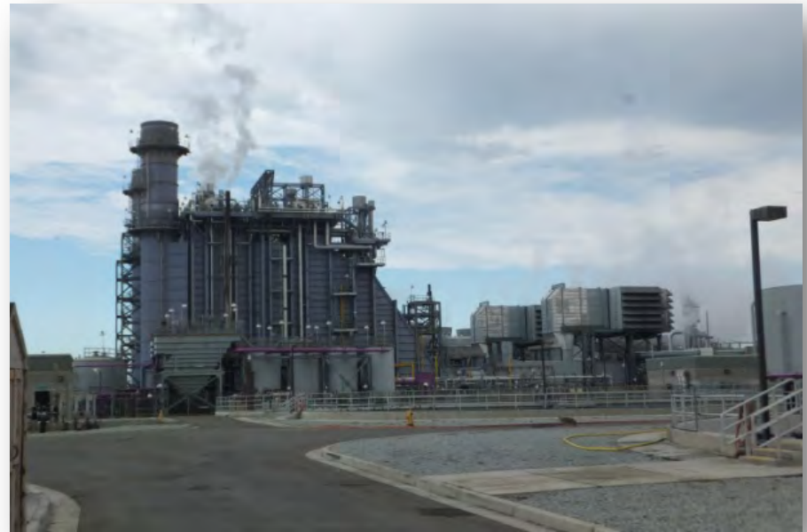
Russell City Energy Center
